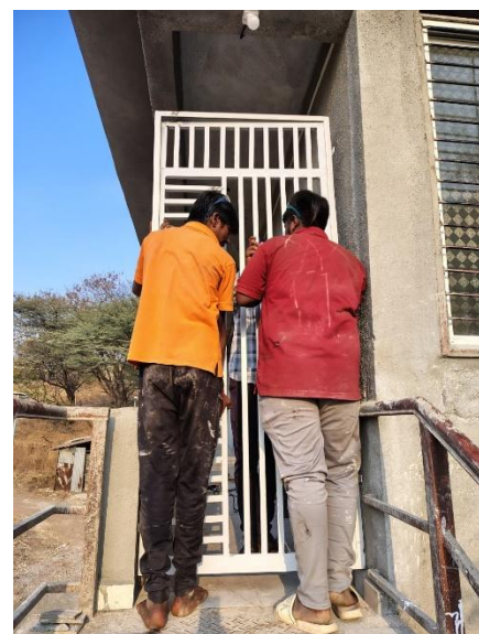
Safety door Installation
