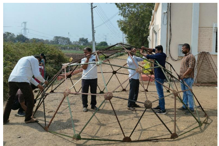
Solar dryer construction
