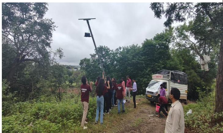
Solar lamp installation by AISSM Institute at campus
