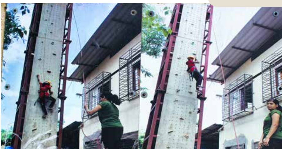
The climbing wall installed by the students of Sumati Balwan School under the IBT program. Interestingly the bulk of the installation work was done by girls @ Sumati Balwan
