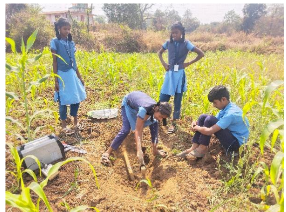
Students of Sangise school repaired pipeline
