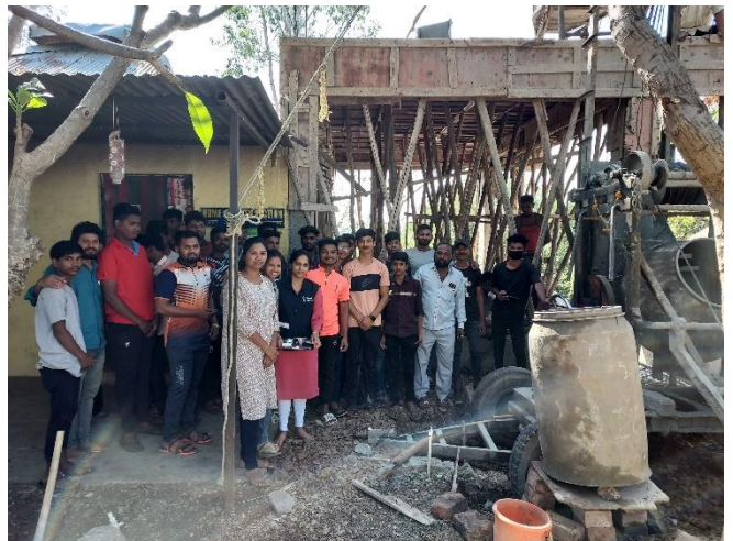
Slab for food lab expansion
