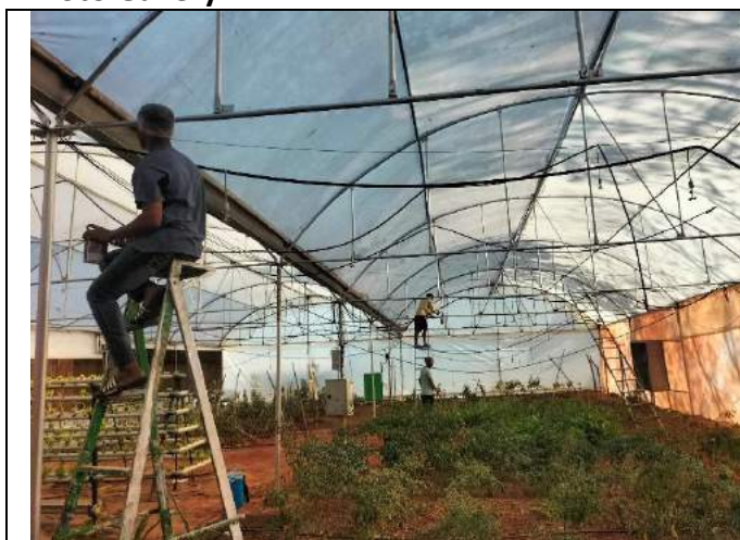
Polyhouse repairing work in progress
