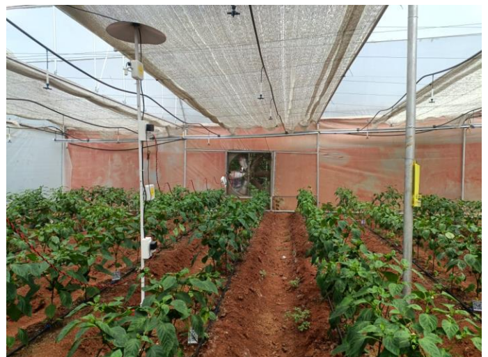
Data Loggers installed inside Polyhouse
