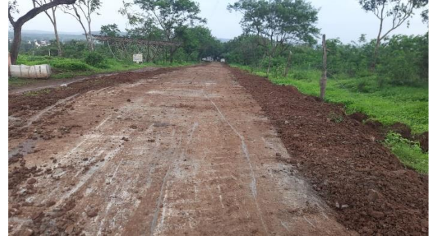
Road completed ( 30 th July )
