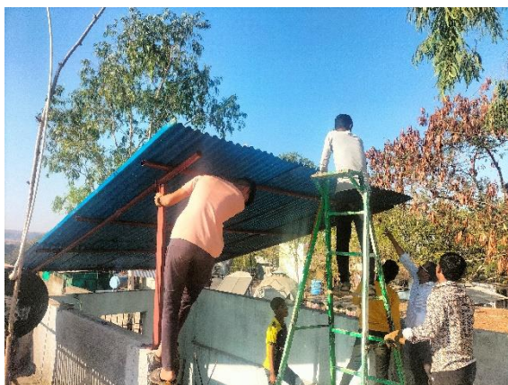
Fabrication of shed
