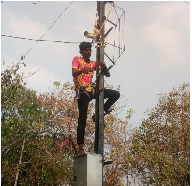
Installation of CCTV camera's on campus
