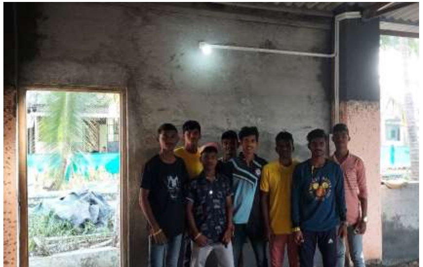
DBRT students completed electrical wiring of community hall
