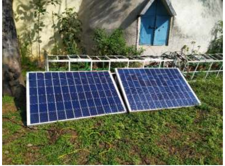
Solar panel was install at DIY during temporary powercut at IIE-JPNC
