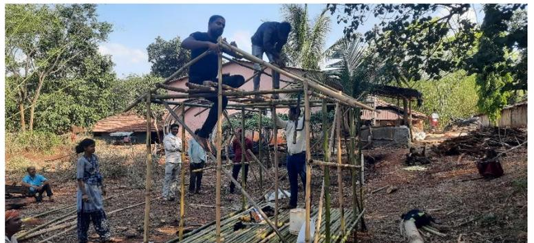
**Poultry cage using bamboo**
