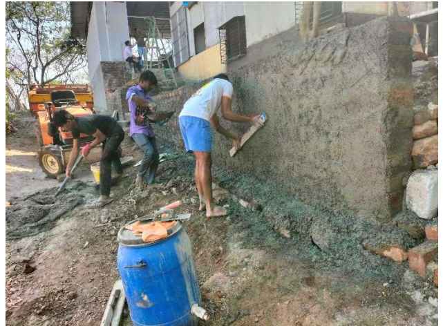
Retaining wall construction
