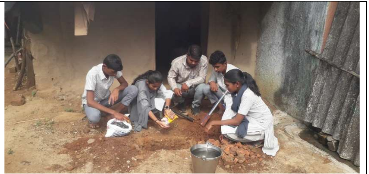
Testing earthing in a village
