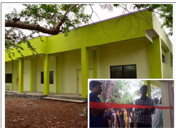
New Classroom / auditorium constructed at Pabal campus
