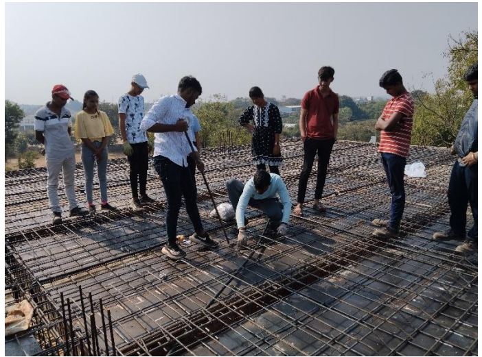
Learning about RCC slab on site
