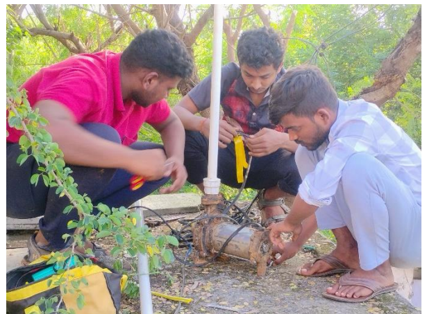
Installing electric motor
