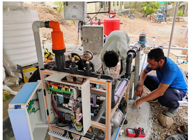
Installation of Fertigation unit
