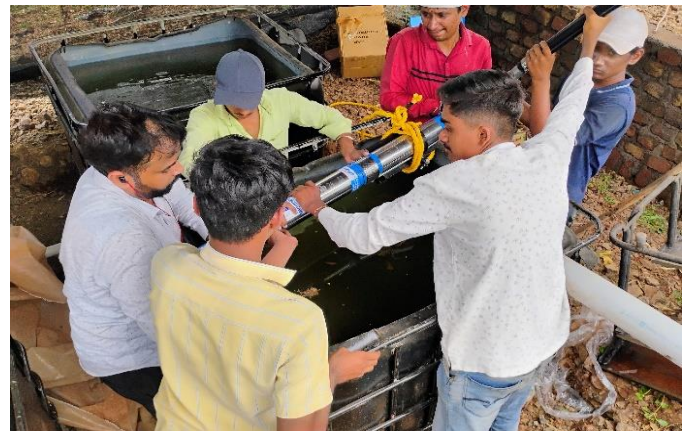
Installing 2Hp pump by DBRT students
