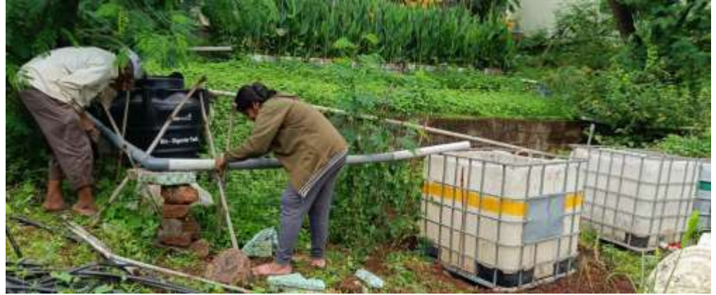
Black water recycling system installation
