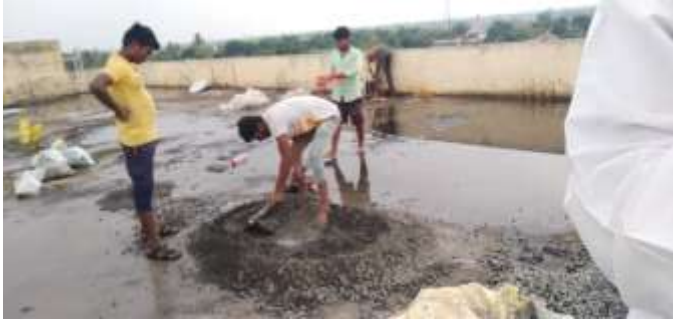
DBRT students preparing cement block for solar panel installation @ Mukhai school
