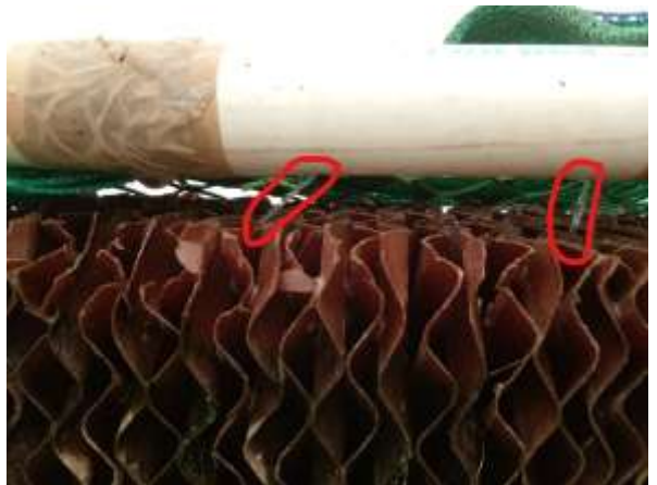
Modification of water distribution holes
