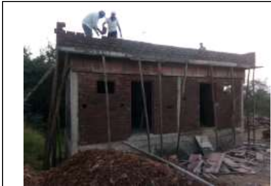
Toilet construction in progress
