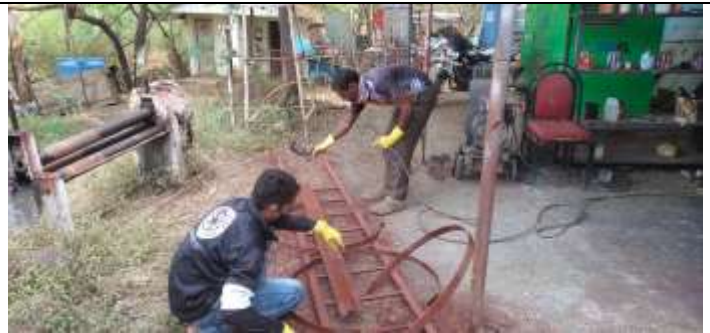
Fabrication of ladder
