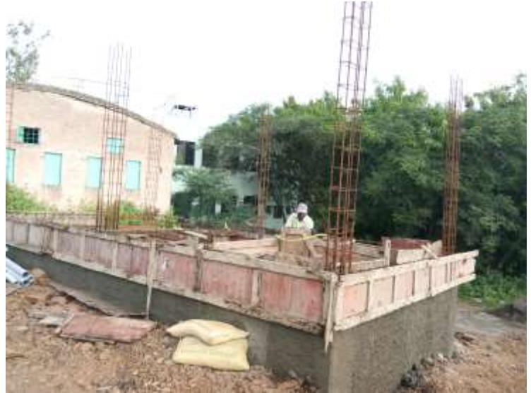
ASHA project : Toilet construction in progress
