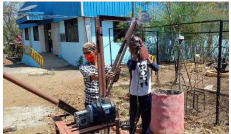
Installing gate at entrance
