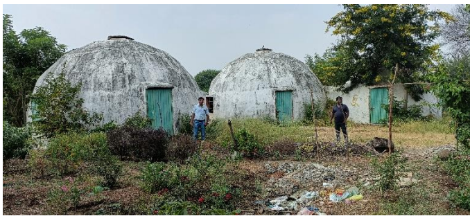
Dome constructed during 1993 Latur Earthquake at Village Gubal. Yogesh Kulkarni visited Gubal on 2nd Nov.
