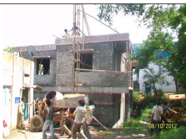
RCC slab work : Staff Quarter
