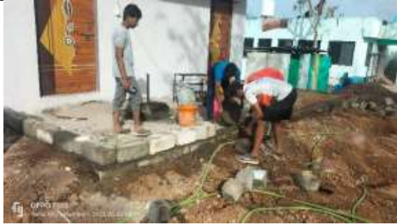
Construction practical : Preparing otta
