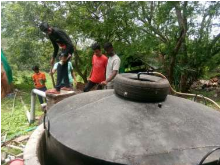
Maintenance of Biogas
