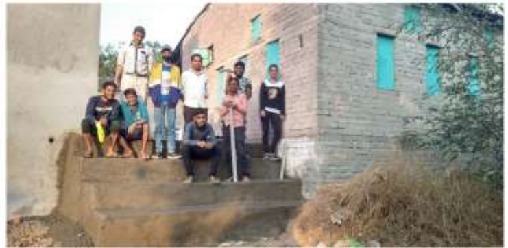
Steps construction for new toilet
