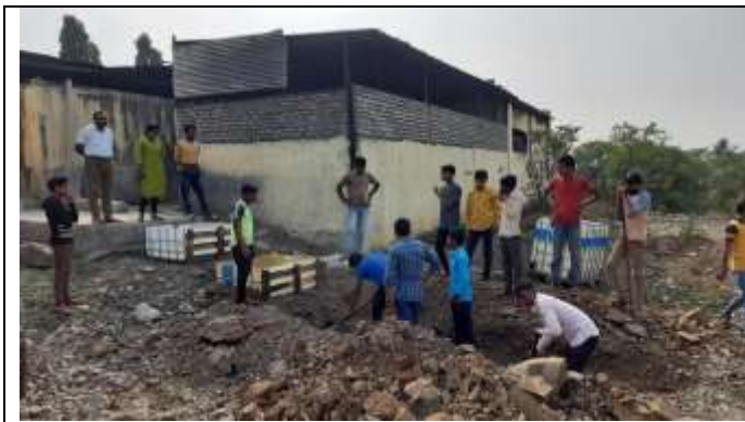
Installing grey water system @ Mukhai School
