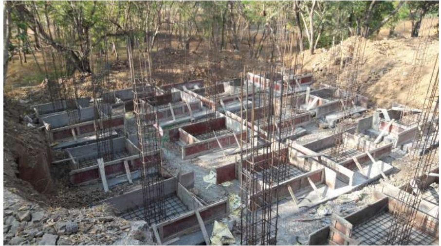
Status of hostel construction
