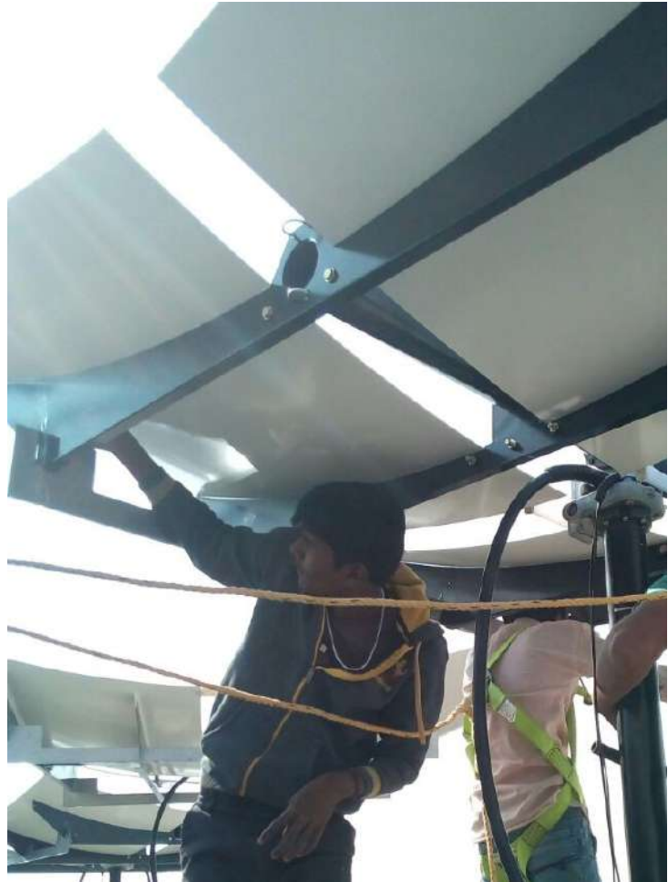
Solar installation Training
