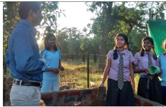
Vermi compost pit construction
