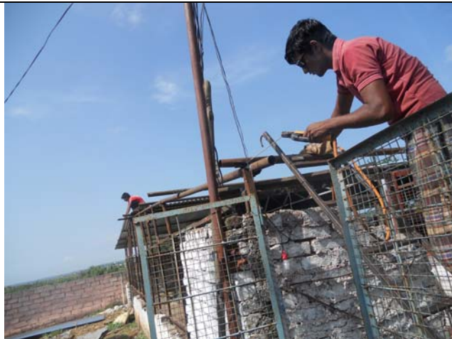
Dairy shed fabrication
