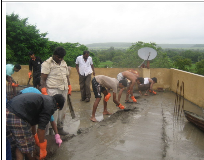
Water proofing of staff quarter : DBRT practical
