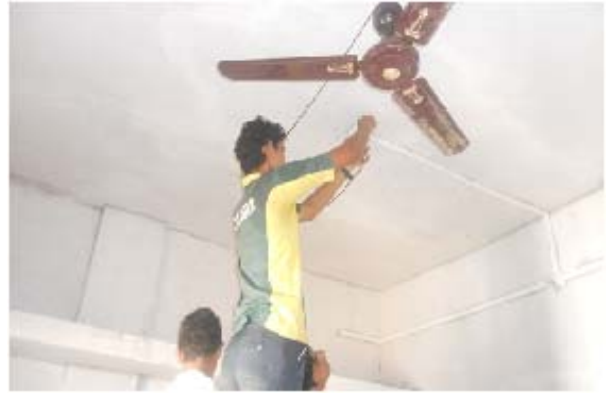
Installing ceiling fan in guest house
