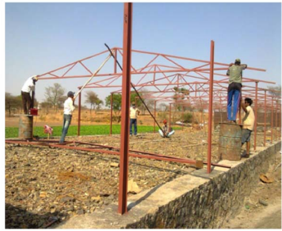
DBRT students did welding of shed at Dhamari
