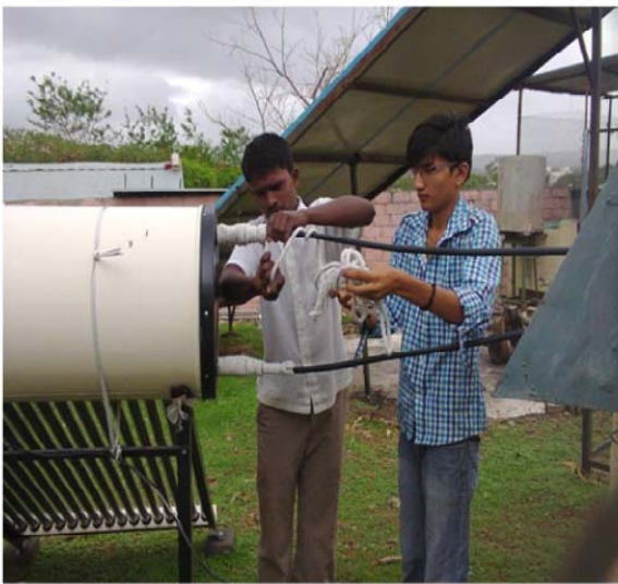
Solar water heater installation
