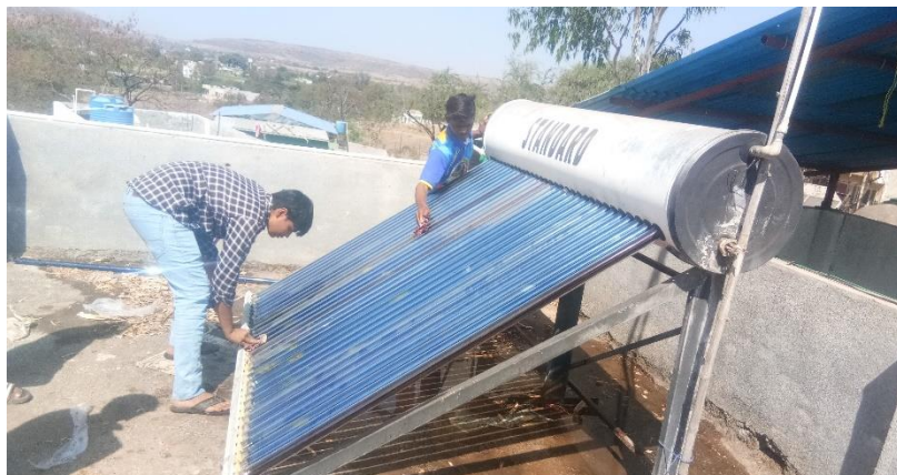
Solar water heater maintenance
