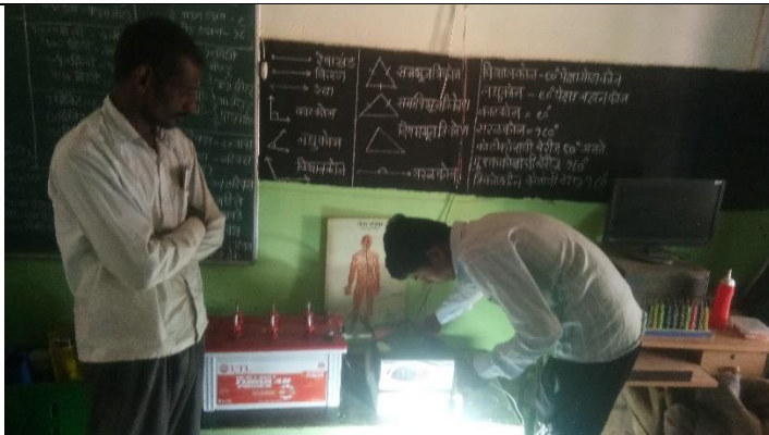
Shramdaan @ ZP High school, Zhodakwadi – Inverter repair
