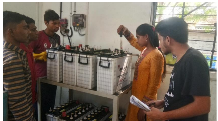
Inverter battery maintenance
