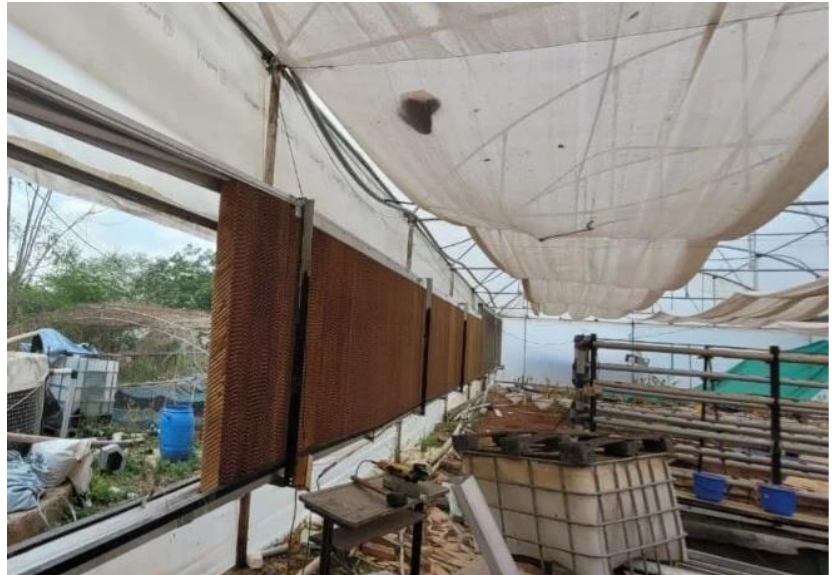
Polyhouse Fan Pad system under construction
