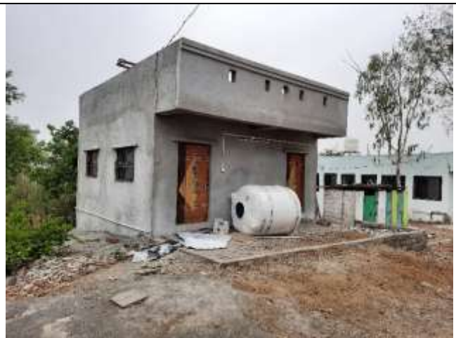
Boy's recreation room towards completion
