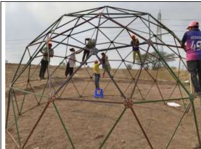
DBRT : Dome nursery construction @ Dhamari
