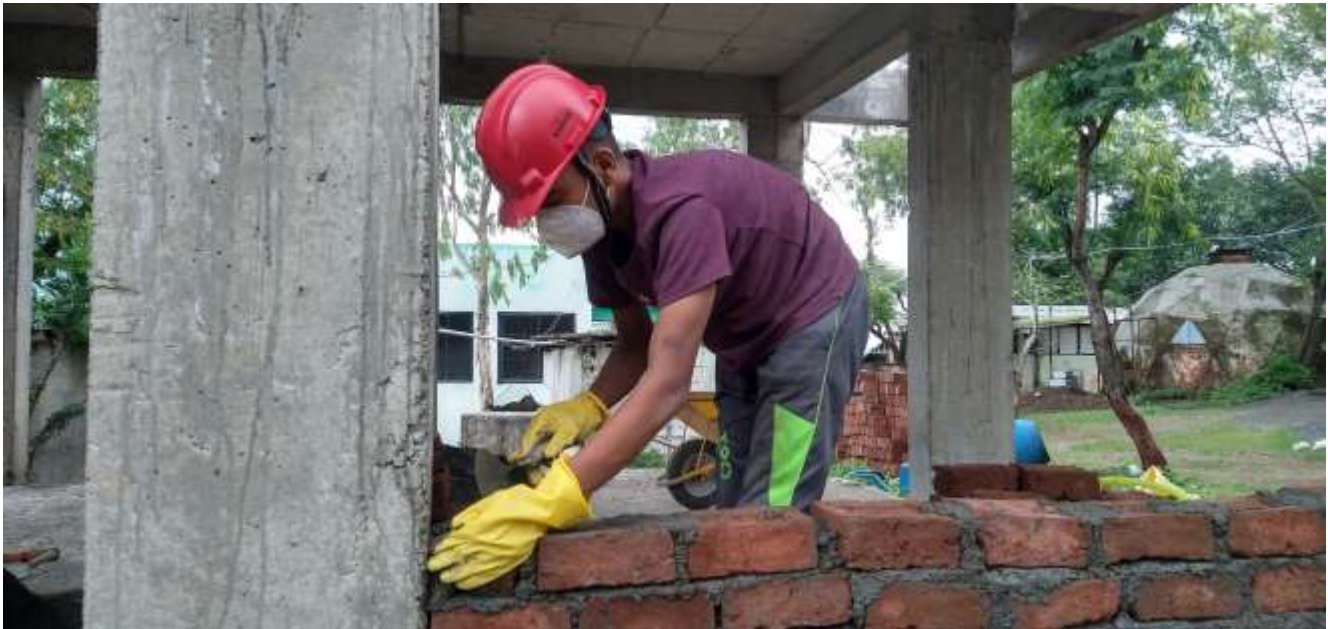
Recreation center construction
