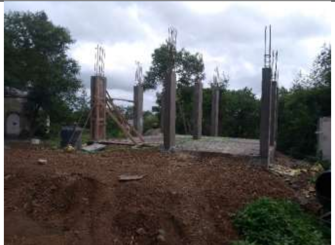
Boys recreation construction status
