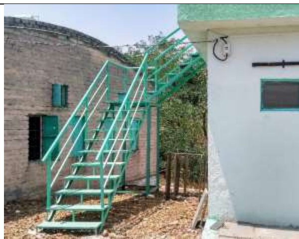
Staircase fabricated by DBRT students
