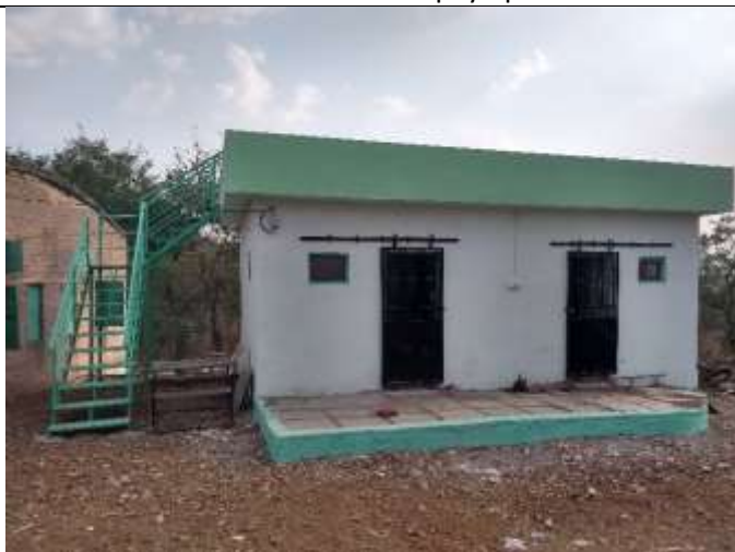
Completed toilet block
