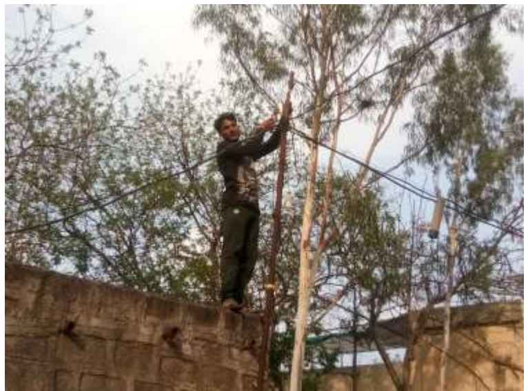
Omprakash working on electric pole
