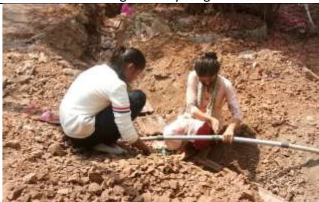
Electric cable laying on campus
