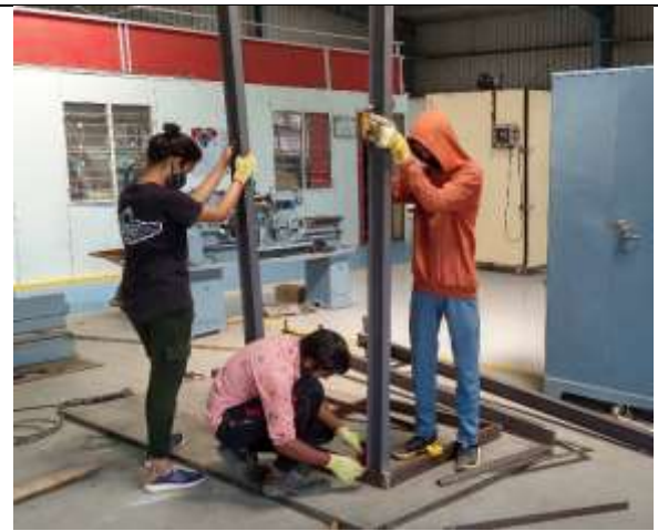
Fabrication of stair case
