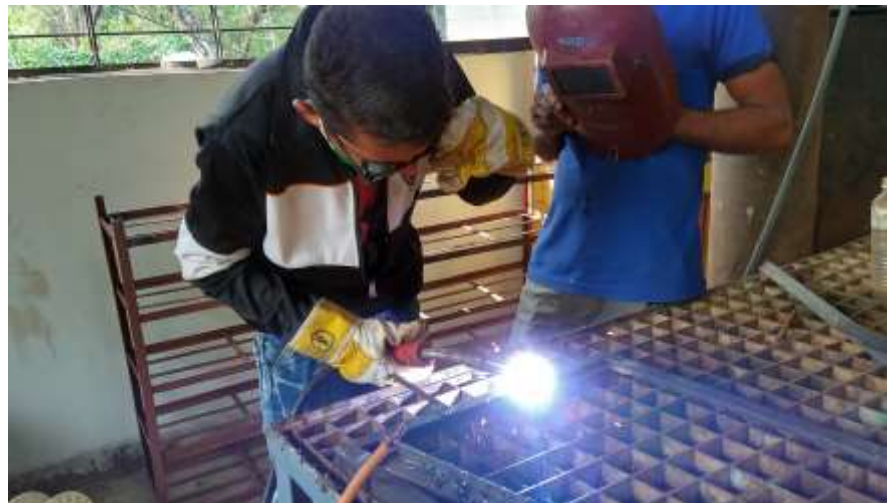
Fabrication of planting structure
