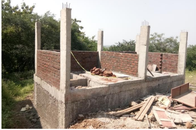
Asha for Education supported Toilet construction status
