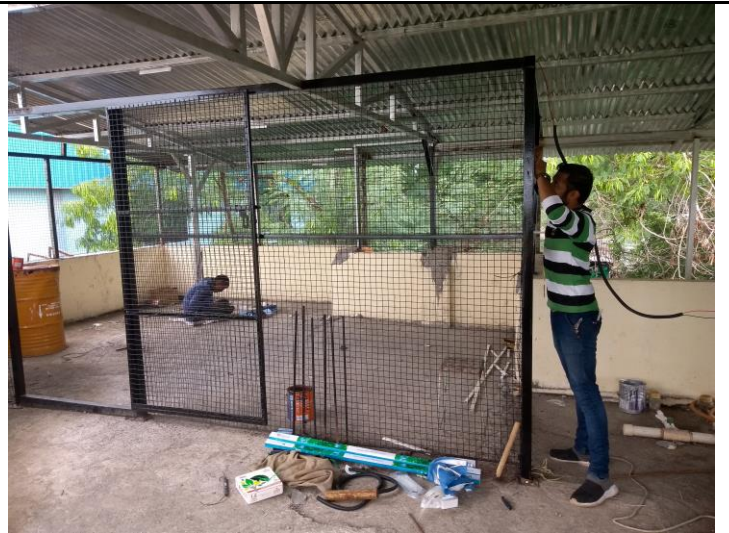
Work in progress : Ladies recreation room
