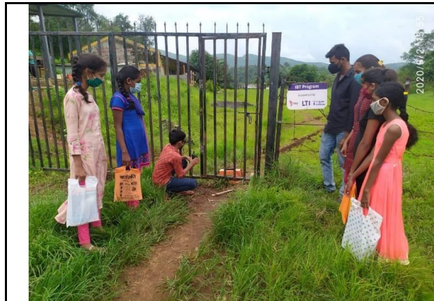
Repairing gate @ Amboli school
