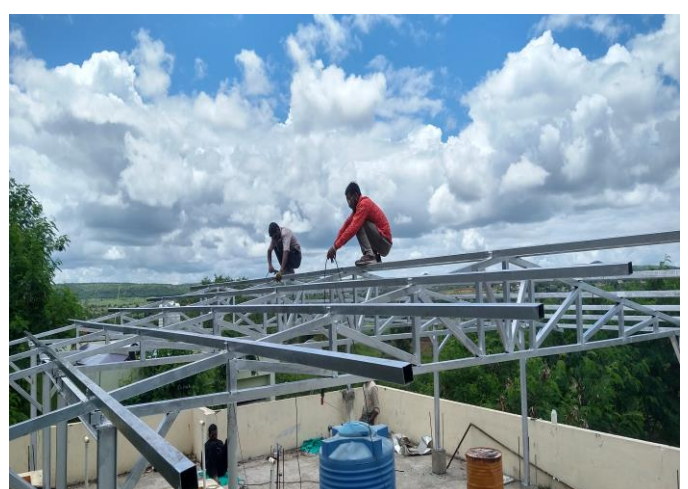
Ladies Hostel shed work in progress.
