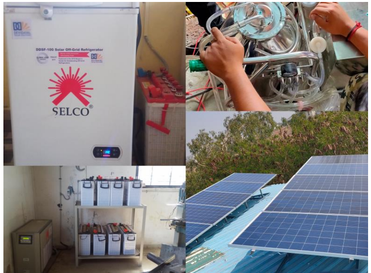
Photo Clockwise – Solar DC Fridge , Milking machine, Solar panel, workshop inverter
