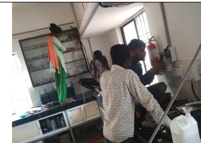
DBRT : Electrical wiring @ Soil Lab
