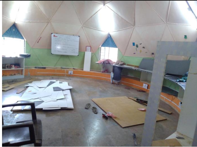
Interior work in progress @ DIY Lab
