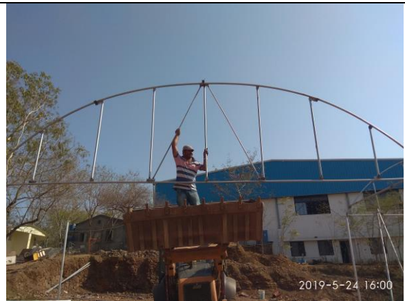
Polyhouse construction in progress
