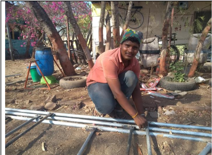
DBRT students fabricated arches for polyhouse
