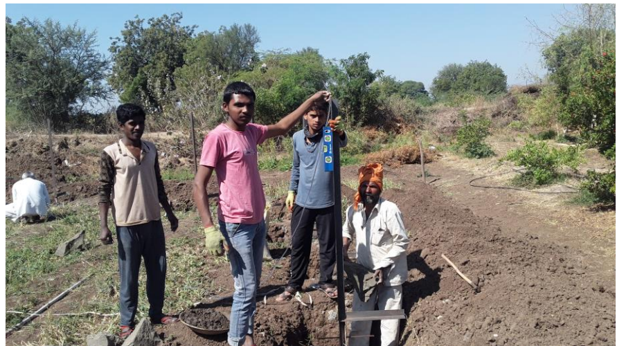
Work on site : Farm Tank
